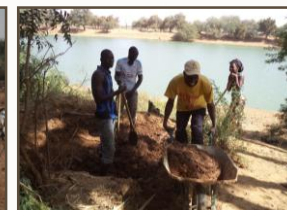
Guede Eco-guards making mud brick for classroom construction
